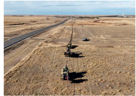
You can see their progress heading east of Lantry.
