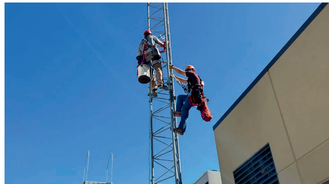
Eric and Andy mount antennae back onto the tower.
