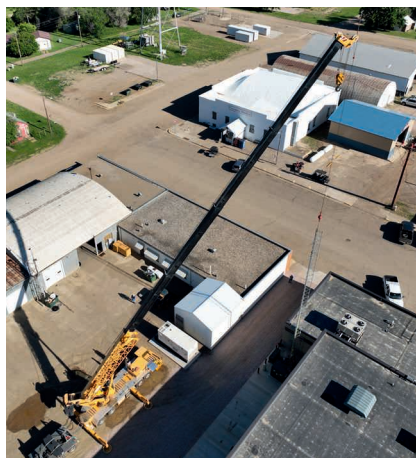
The operator deftly swung the tower from the old base to the new.
