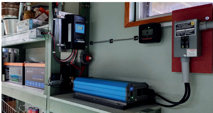
The hardware and storage that enables the Velsko's solar array to stay off grid
