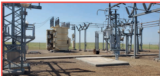
The concrete pad in the foreground will be the home for the new WAPA transformer serving the growing needs of Eagle Butte and surrounding areas.
