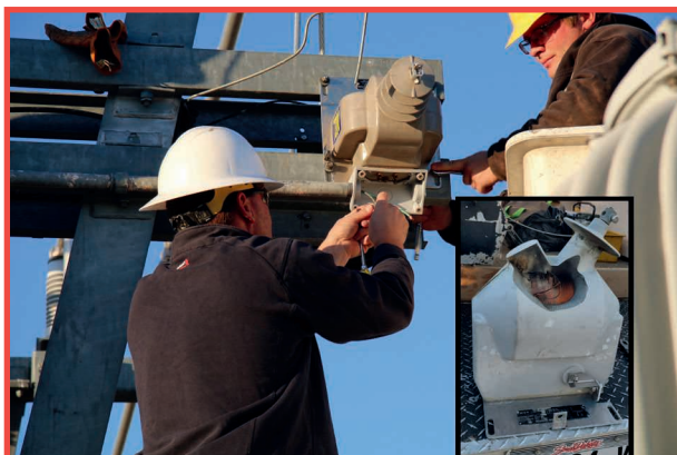
Josh and Troy replacing damaged voltage transformer at the Timber Lake sub. The inset photo shows damaged equipment.
