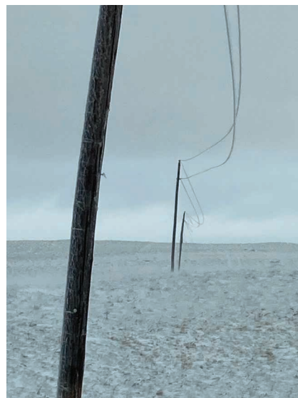
High winds and ice placed a lot of strain on the power lines. Photo by Staking Foreman Hunter Smith
